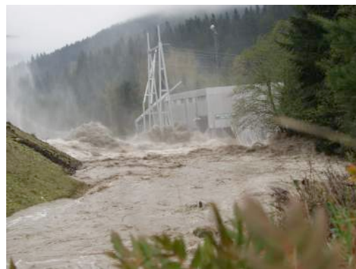
Canal Water Inundating Powerhouse and Local Highway
