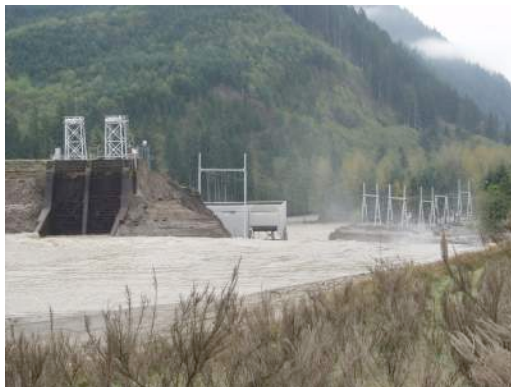
Canal Water Escaping Embankment Breach
