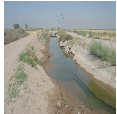
Liquefaction caused Undulating Surface along the Bank of the Canal in Unit 11
