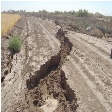
Large Ground Fissure Running Across the Road Near the Hardy River
