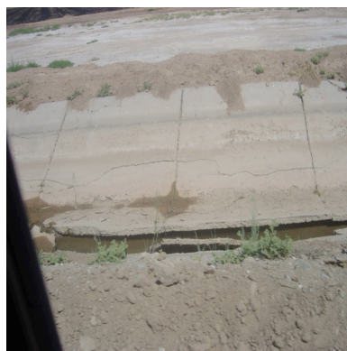
Liquefaction-induced Lateral Spreading Caused Flattening of the Side Slopes
