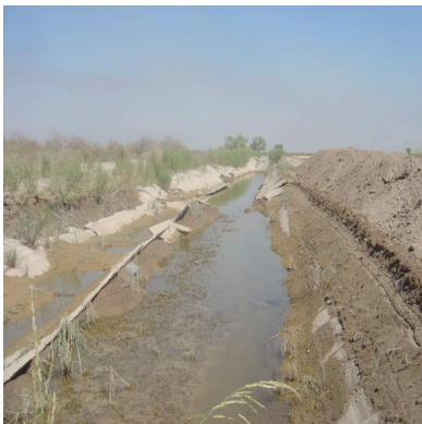
Lateral Spreading Caused the Concrete Panels to Slide and Buckle at the Toe in Unit 11
