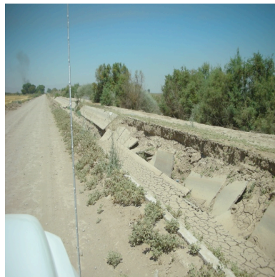
Sliding of Land Mass and Cast-in-place Concrete Liner Panels
