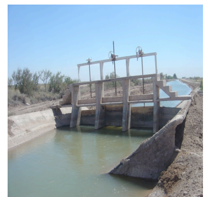
Lateral Displacement of Concrete Side Panel, Causing Tilting of Flood Gate in Unit 12
