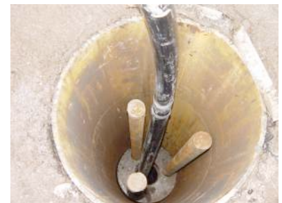
Tremie Grouting Finished Caisson
