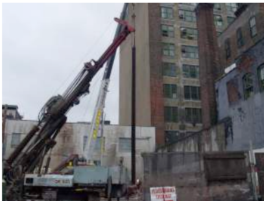
Installing Reinforcing Cage Inside Caisson
