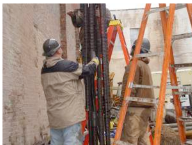
Coupling Sections of Rebar Cage
