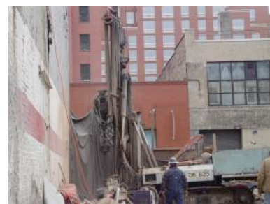
Drilling Small Diameter Caissons
