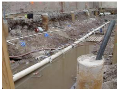
Dewatering around Caisson Caps
