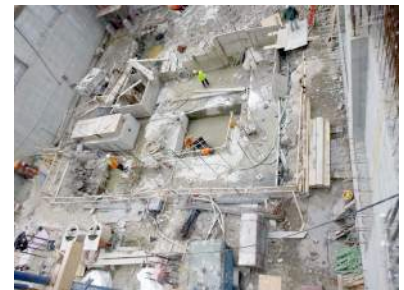
Nearly Complete Foundation
