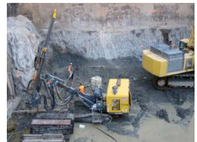
Line Drilling and Rock Removal
