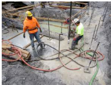
Tiedown Anchor Inspection
