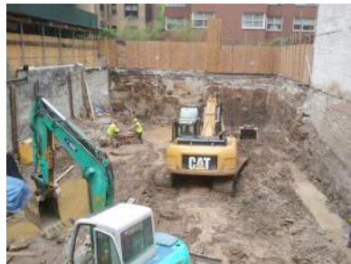
Excavation & Foundation Prep Prior to Underpinning
