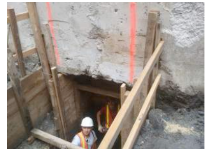
Underpinning in Progress
