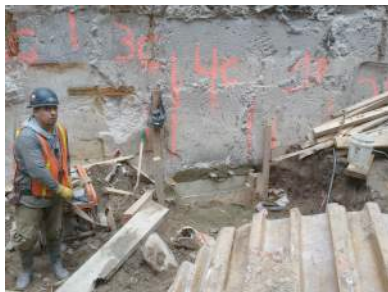
Underpinning of Building to the West
