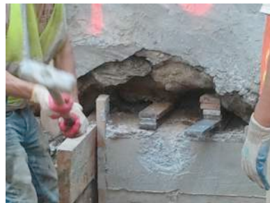
Steel Plates and Wedges at top of Underpinning
