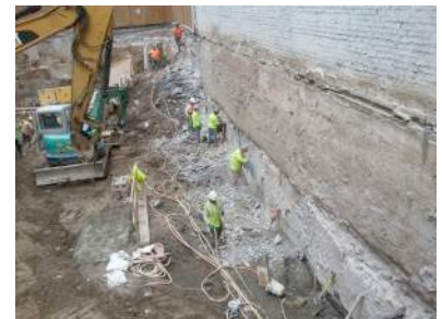
Foundation Prep prior to Underpinning
