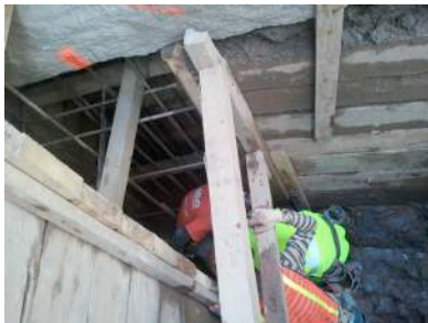
Underpinning at SE corner of site
