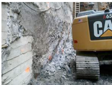
Neighboring Building Transitions from Rock to Concrete Underpinning
