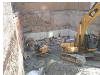
Excavation for New Footings at Completion of Underpinning and SOE
