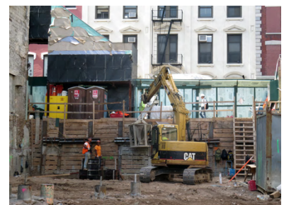
Soldier Beam & Timber Lagging Wall
