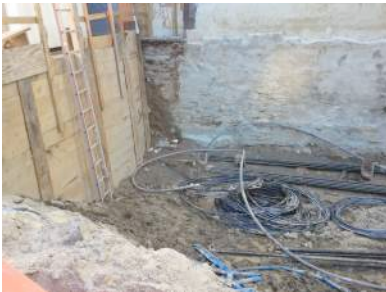
Soldier Beam & Lagging Walls Along Open Lot Lines
