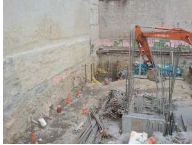
Underpinning & Bracing of Adjacent Structures
