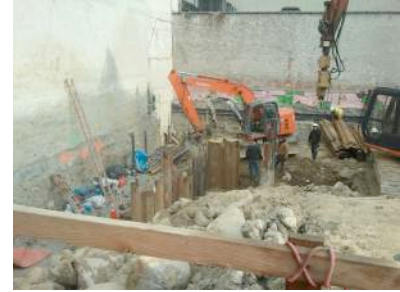
Steel Sheetting for Core Foundations
