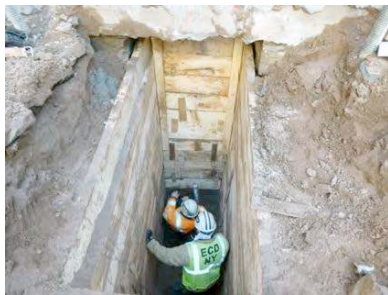
Titan Pile at Bottom of Underpinning Pit
