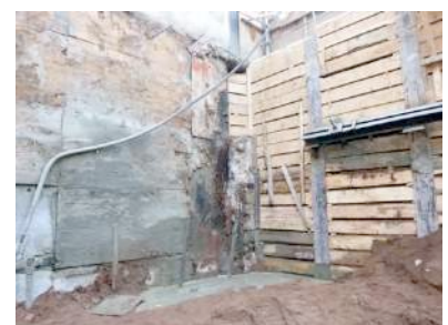
Excavation in Progress
