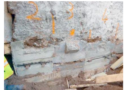
Steel Plates and Wedges to Transfer Foundation Loads
