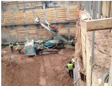
Drilling Tiebacks at Second Wale
