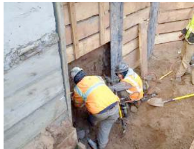
Installation of Lagging Boards
