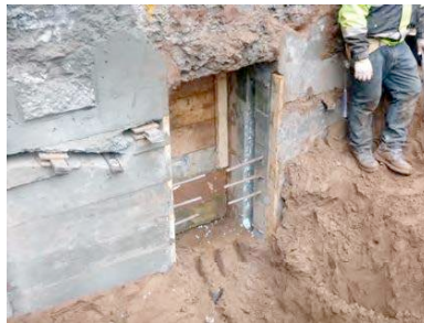
Continuous Internal Reinforcing of Underpinning Concrete
