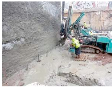
Installation of Titan Piles Prior to Underpinning
