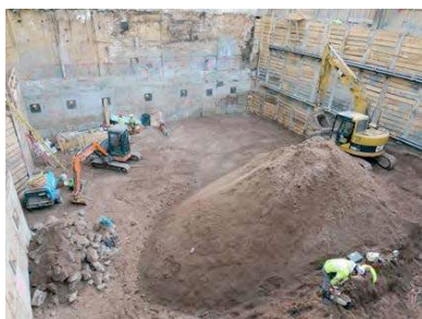
Nearly Complete Excavation- Preparation for Mat Foundation
