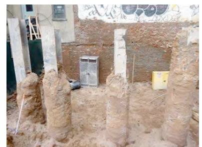
Soldier Pile Installed in Pre-drilled Holes with Grout Backfill
