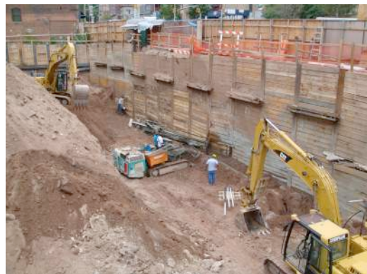
2nd Level Tieback Installation of Soldier Beam and Timber Lagging Wall
