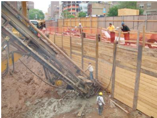
Tieback Installation of Soldier Beam & Timber Lagging Wall
