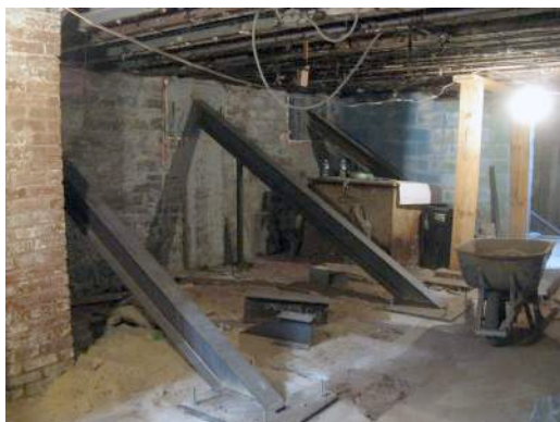
Temporary Bracing inside East 4th St Building
