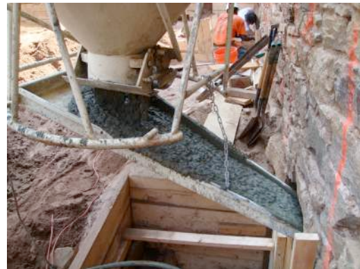
Concrete Pour for Underpinning of Building on East 4th St
