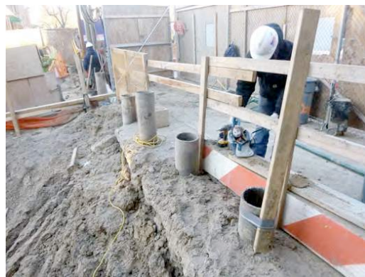
Drilled Soldier Piles at Property Line
