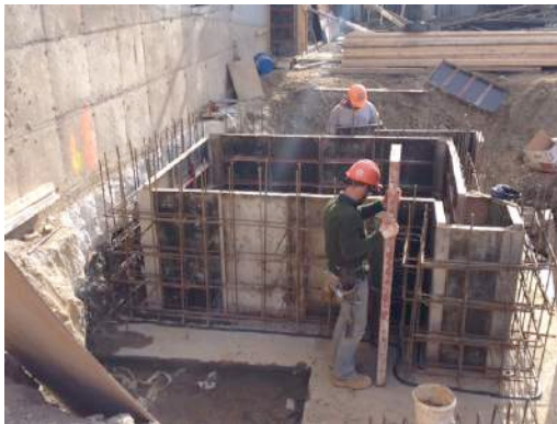
Shallow Foundation on Bedrock
