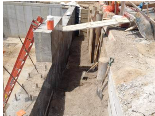
Partial Backfill Outside Foundation Wall
