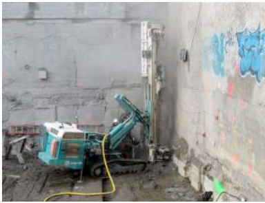
Caisson Installation after Underpinning
