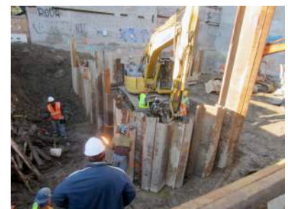
Sheet Pile Installation for Second Level Excavation
