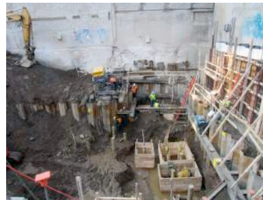
Caisson Cap Construction at Second Level Excavation
