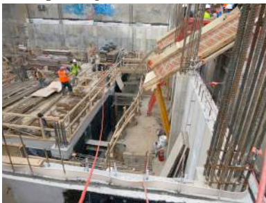
Backfilling Second Level Foundation Walls
