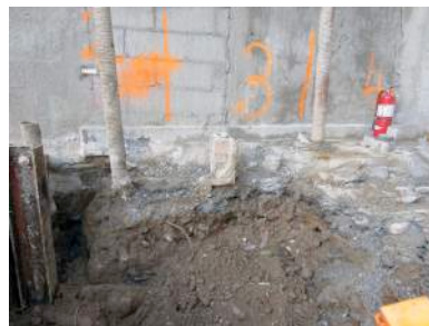
Installation of Titan Piles Prior to Underpinning
