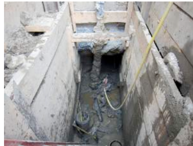
Underpinning Pit with Titan Pile
