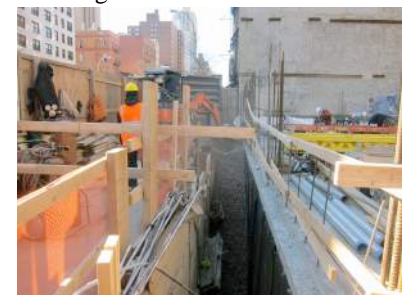
Backfilling First Level Foundation Walls
