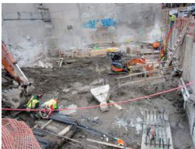
First Level Excavation after Underpinning
