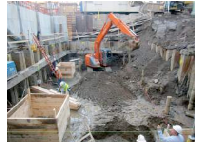
Excavation Inside Second Level Sheetting
